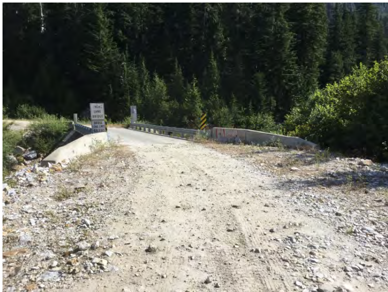
Approach from Left Bank when facing downstream
