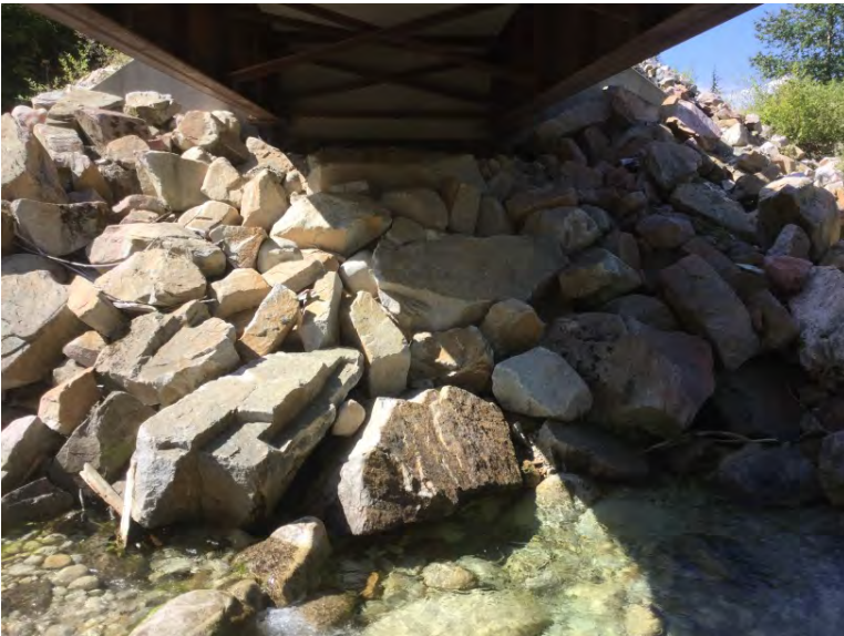
Left Bank Abutment when facing downstream
