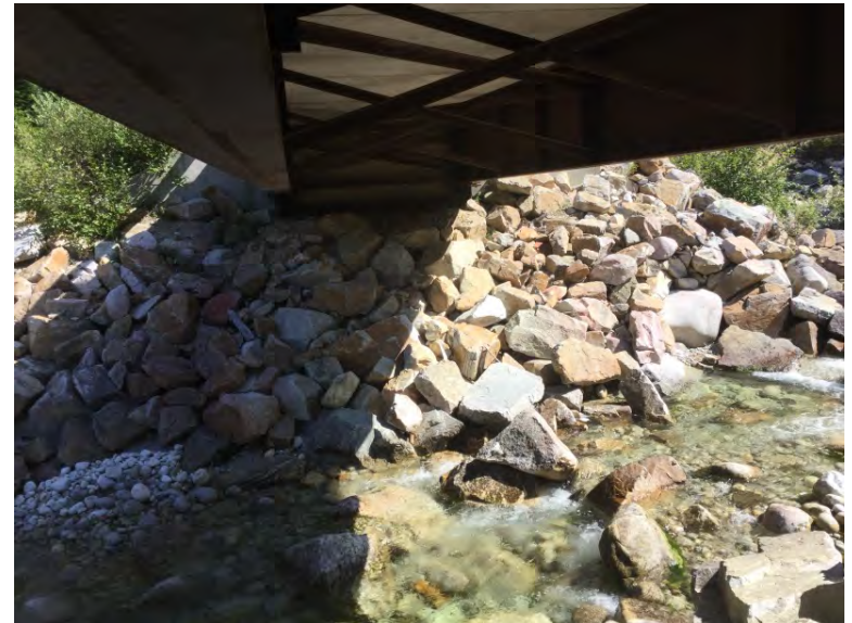
Right Bank Abutment when facing downstream
